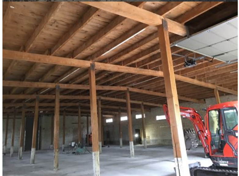
Photo 3: Existing structure: Southeast area of existing building.
