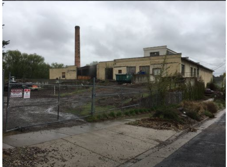
Photo 2: Street view: Looking south toward project. Temp fence installed to discourage entrance.
