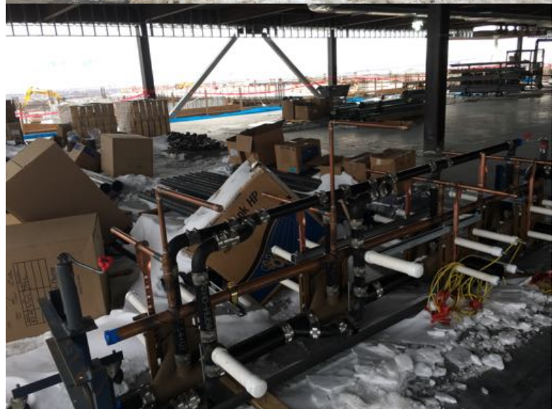
Photo 3: Main floor: Plumbing core for restrooms is on-site. Notice slab is poured.
