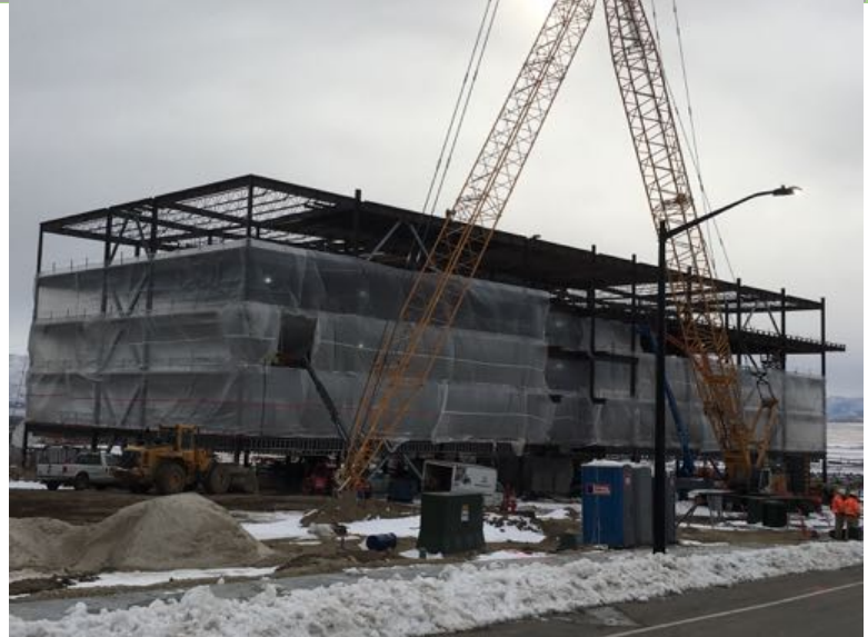
Photo 1: Street view: Structural steel in progress through fifth floor.
